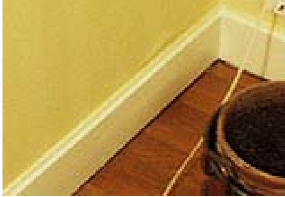
Detection and visualization of Infiltration / Exfiltration. Air leakage through the gap between the wall and the floor.
